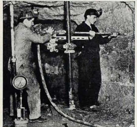
Phil Blazovic (r) AK, preparing to drill a hole for blasting.
